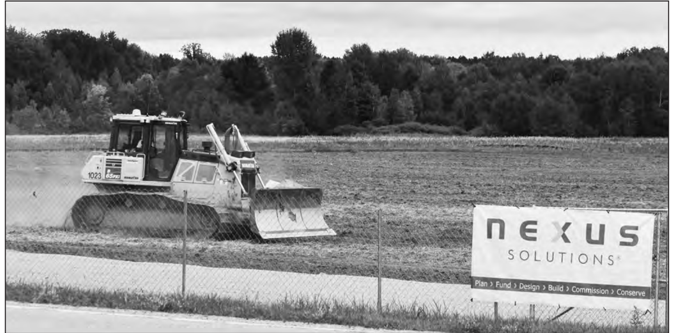
A bulldozer moves soil Sept. 18 at the Oconto Falls Middle School construction site. The public is invited to the formal groundbreaking ceremony for the project on Sept. 27.
