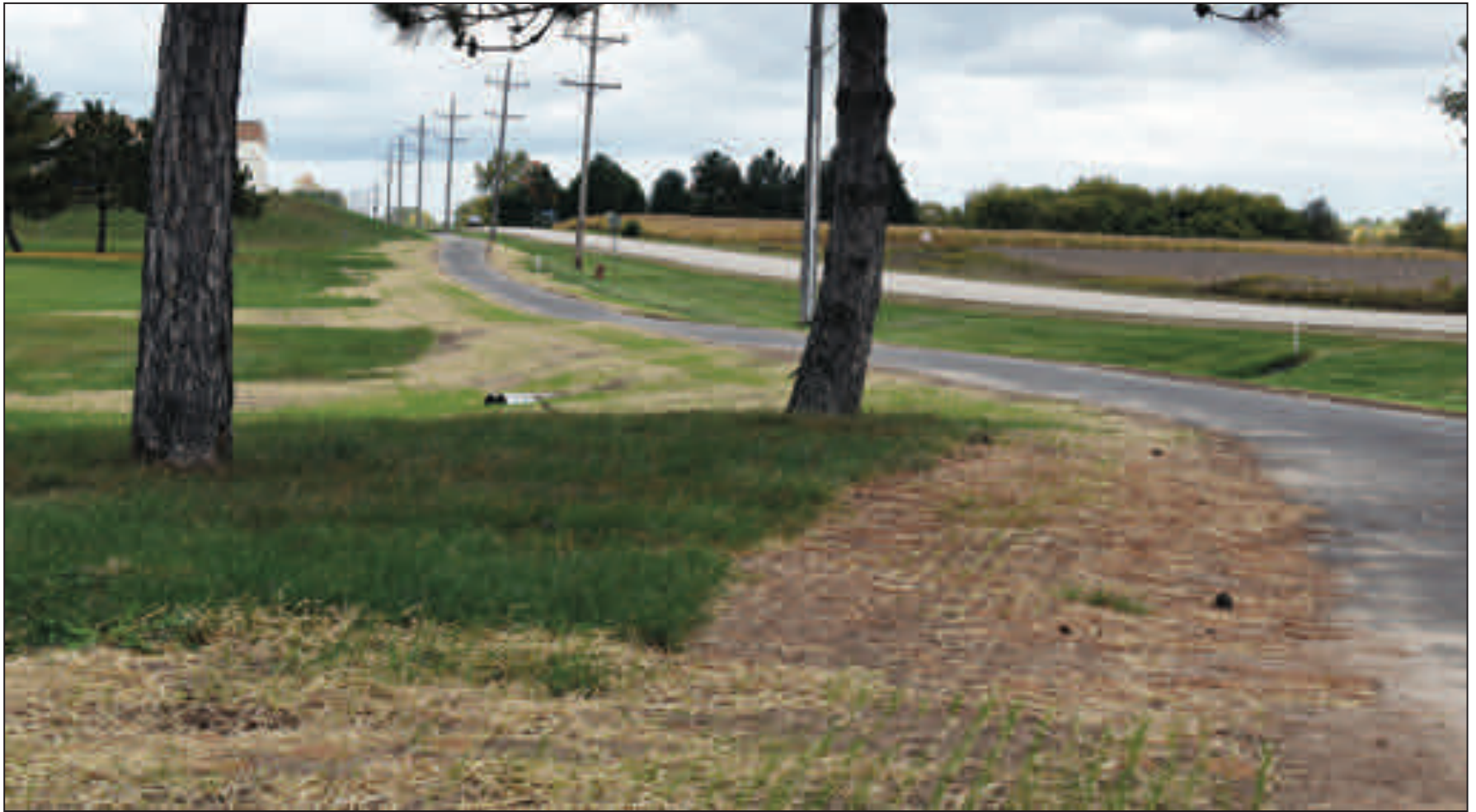
The newly completed segment of the Panther Path walking trail runs from Oconto Falls High School along County Road I to Marie Volk Drive and Oconto Falls Elementary School. WARREN BLUHM | NEW MEDIA
