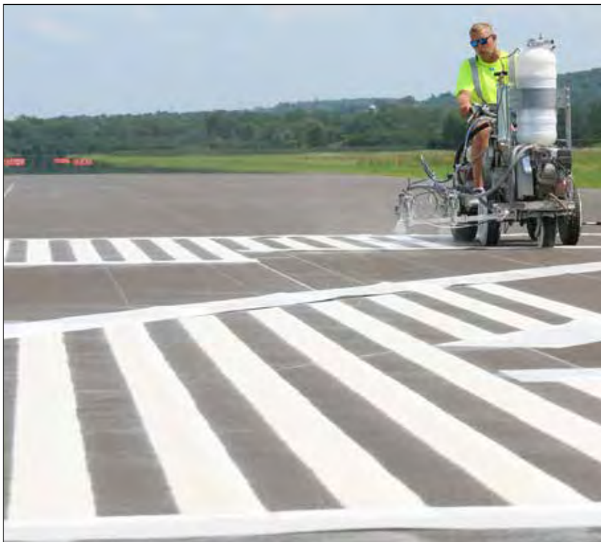
Tony Crawford, Grafton, follows a carefully plotted pattern as he sprays the informational markings on the rebuilt Runway 1230 at Shawano Municipal Airport. CrowleyConstruction, Wauwatosa, was hired to place the markings.
