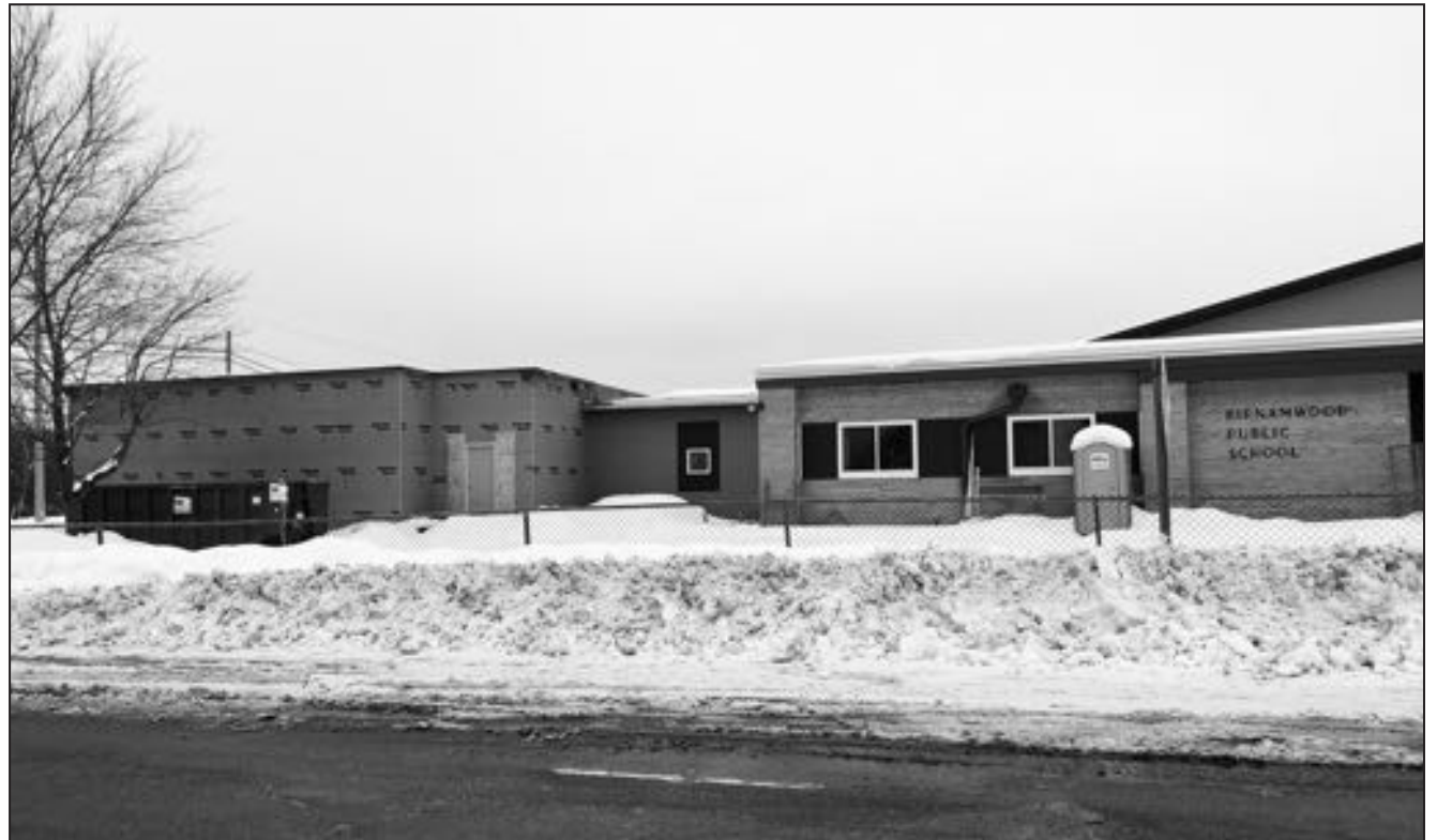
Two new 1,200-square-foot classrooms at Birnamwood Elementary-Middle School are ready to be drywalled. Brick will be added to the exterior this spring. MIRIAM NELSON | NEW MEDIA
