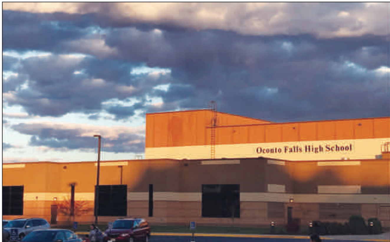
The sun breaks through and illuminates Oconto Falls High School just before sunset on an otherwise cloudy day.
