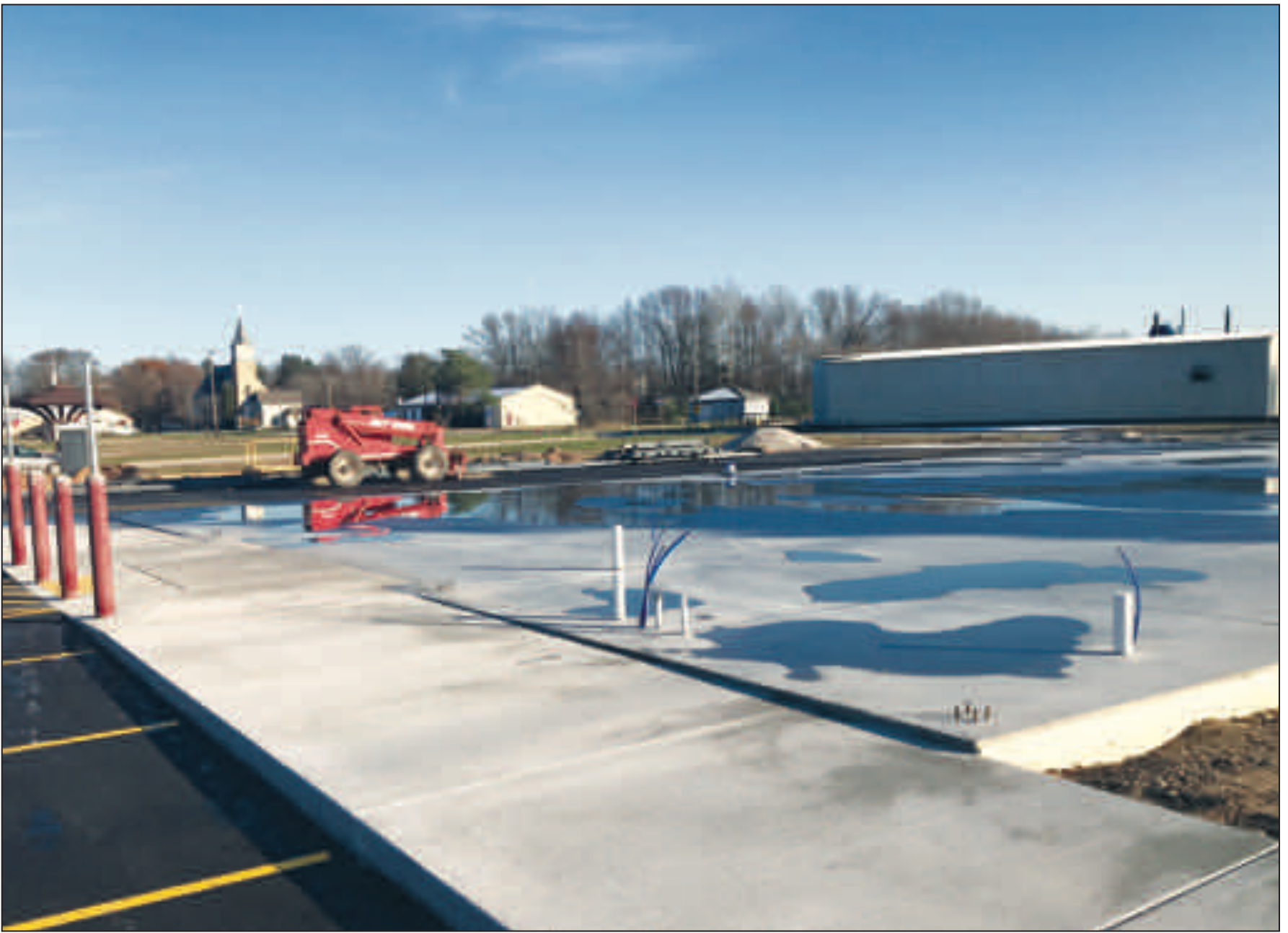
The parking lot is in place, and the concrete slab is ready for construction of the new Dollar General store at 611 E. Main St. in Suring.
