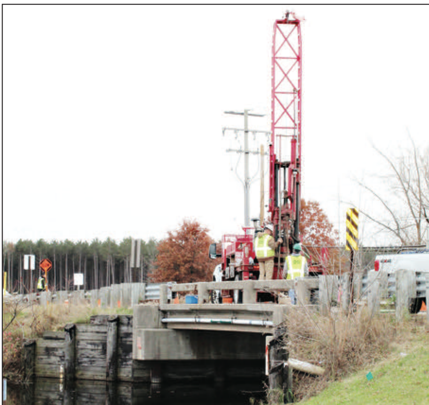
An Intertek PSI crew collects soil samples on Wednesday on the County Road HHH bridge over Shawano Creek, known locally as The Channel. The bridge is slated for replacement in 2022, and the Shawano Area Waterways Management organization is encouraging residents to request a wider, higher bridge.
