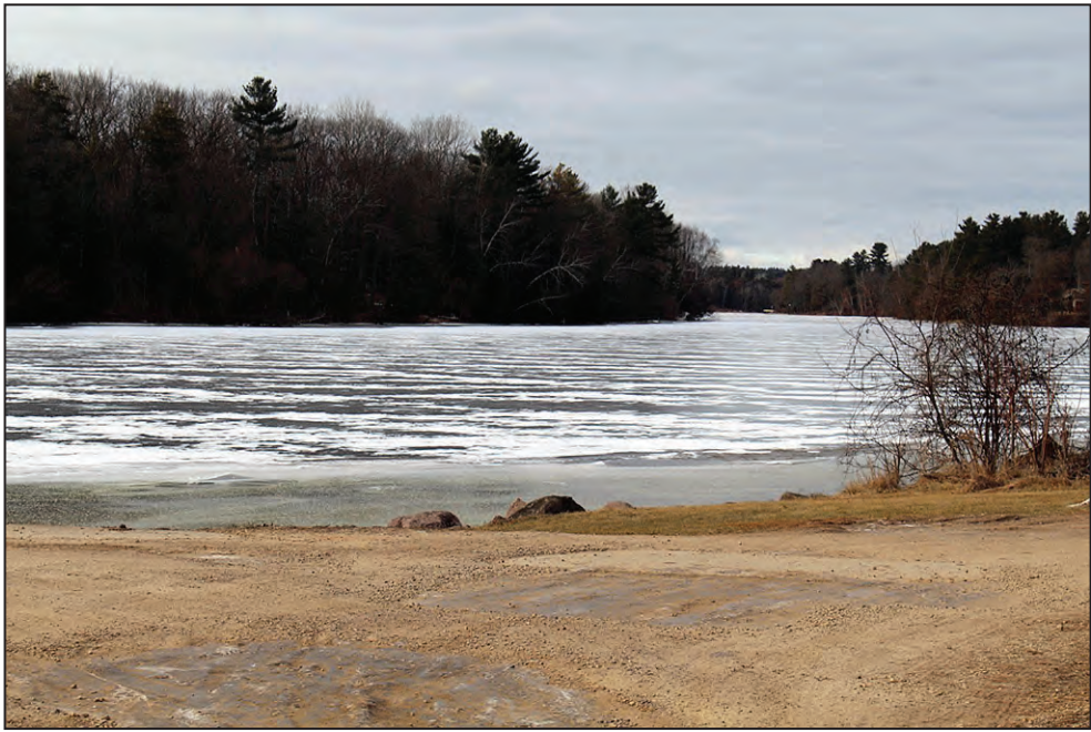
A generator failure at the Balsam Row Road Dam will cause unstable water levels north of the dam for the rest of the winter. Residents are urged to not go on the ice north of the dam, as changing water levels can lead to cracks in the ice. Officials are weighing their options regarding repairs to the dam.
