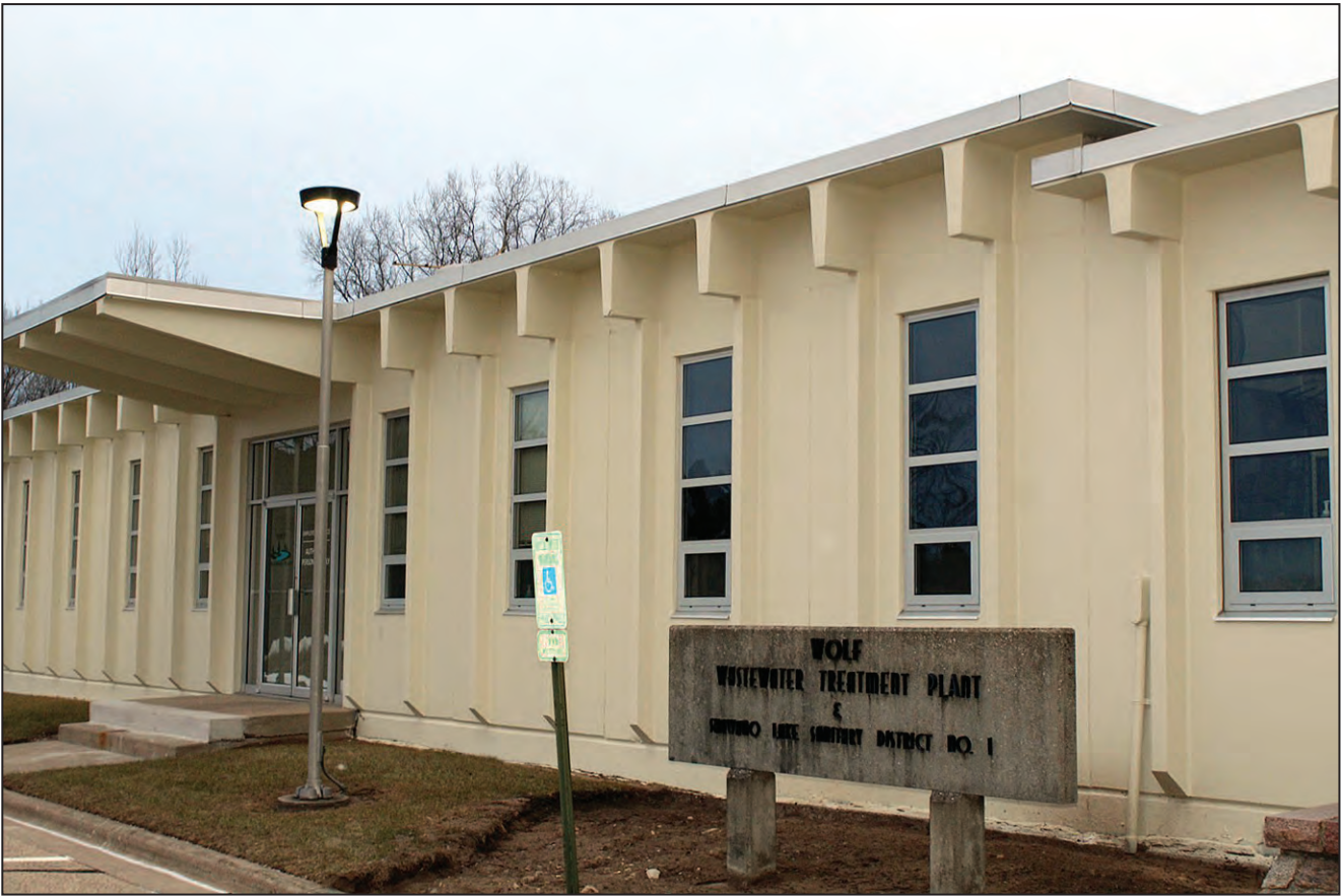
The Shawano Lake Sanitary District is a water and sewer utility and wastewater treatment facility servicing the Shawano Lake and surrounding areas. It employs 11 people who monitor, maintain and administer its operation.
