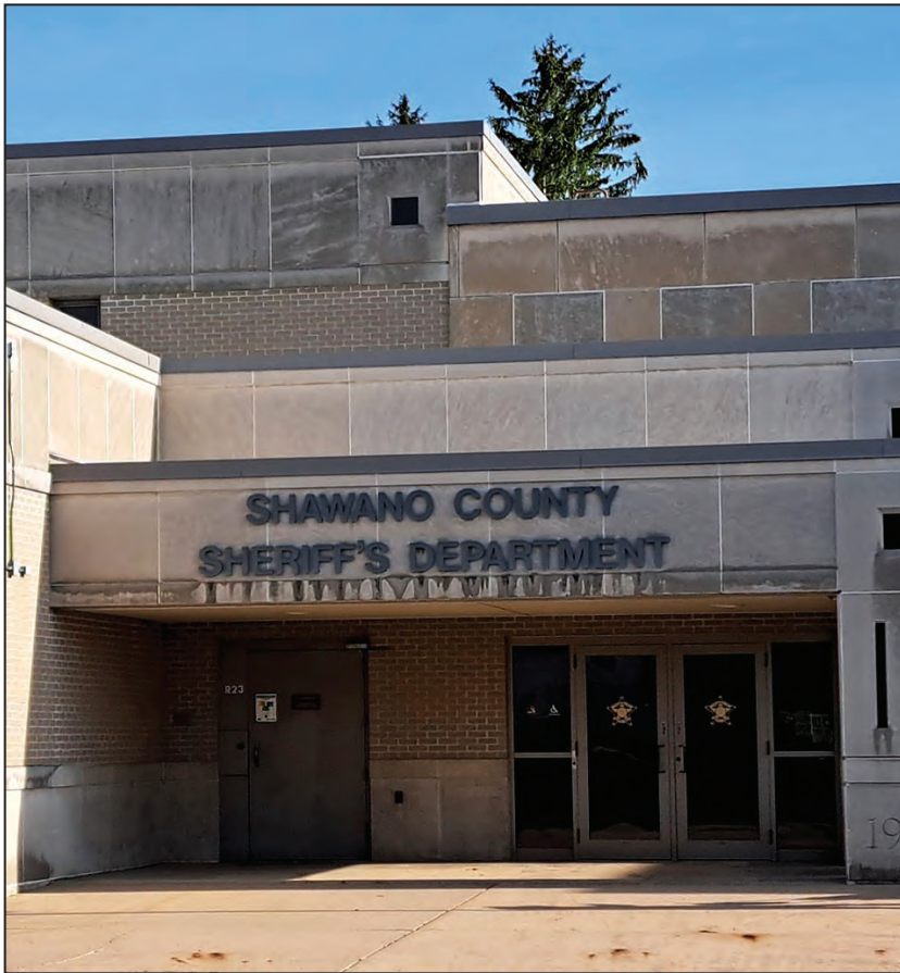
The Shawano County Sheriff's Department and jail building will be among the projects studied by an ad hoc building committee. The committee is tasked with recommending a master plan for county-owned buildings. The plan will include recommendations to construct new buildings, remodel existing ones, maintain existing buildings without remodeling them or any combination. KEVIN PASSON | NEW MEDIA
