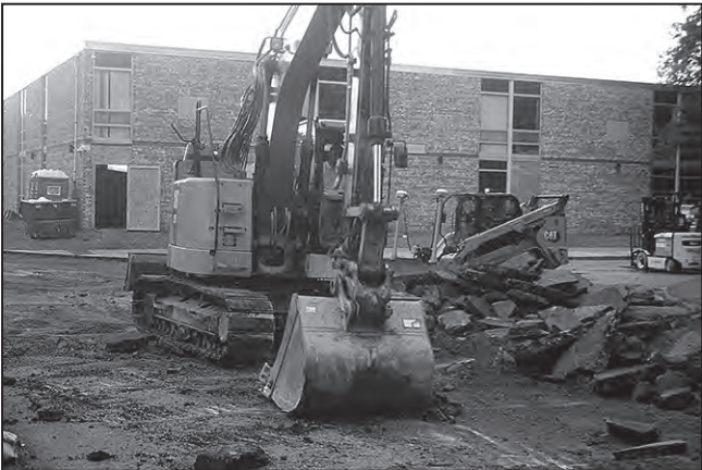
Heavy equipment clears out some asphalt July 24 in front of Olga Brener Intermediate School as part of the construction work that includes adding district office facilities at the school. The current district offices are going to be where new athletic facilities are going in at Shawano Community High School. Other work going on at Olga Brener includes roughing in interior walls and the installation of new lighting throughout the school. Projects at the other schools include the installation of new rubber roofing at Shawano Community Middle School, as well as repairing cracked bricks and installing a new concrete sidewalk at Hillcrest Primary School. Construction projects at SCHS will begin later in August, with a groundbreaking ceremony at 10 a.m. Aug. 26. LEE PULASKI | NEW MEDIA
