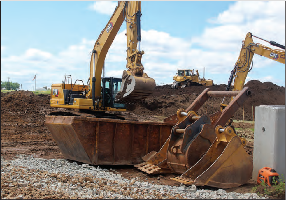
Construction work has already begun for the Bear Trail Crossing apartment complex on state Highway 29, even before the July 17 groundbreaking. Once complete, there will be 48 two-bedroom apartments that will help ease demand for housing in the village of Bonduel.
