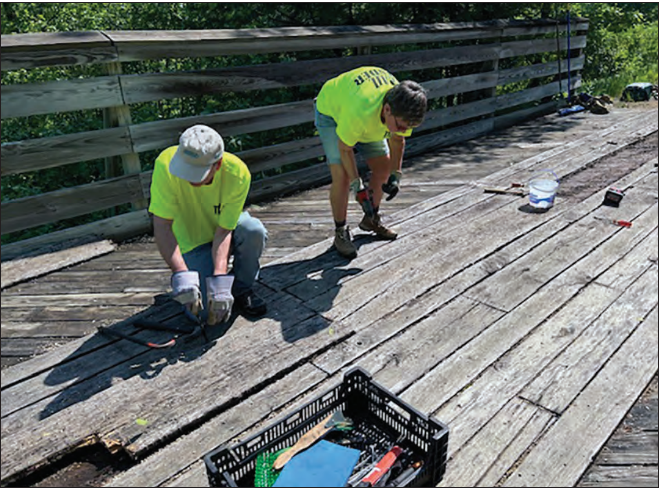
Lee Bengston and Christine Bartz work on bridge repairs along the Mountain-Bay State Trail west of Shawano.
