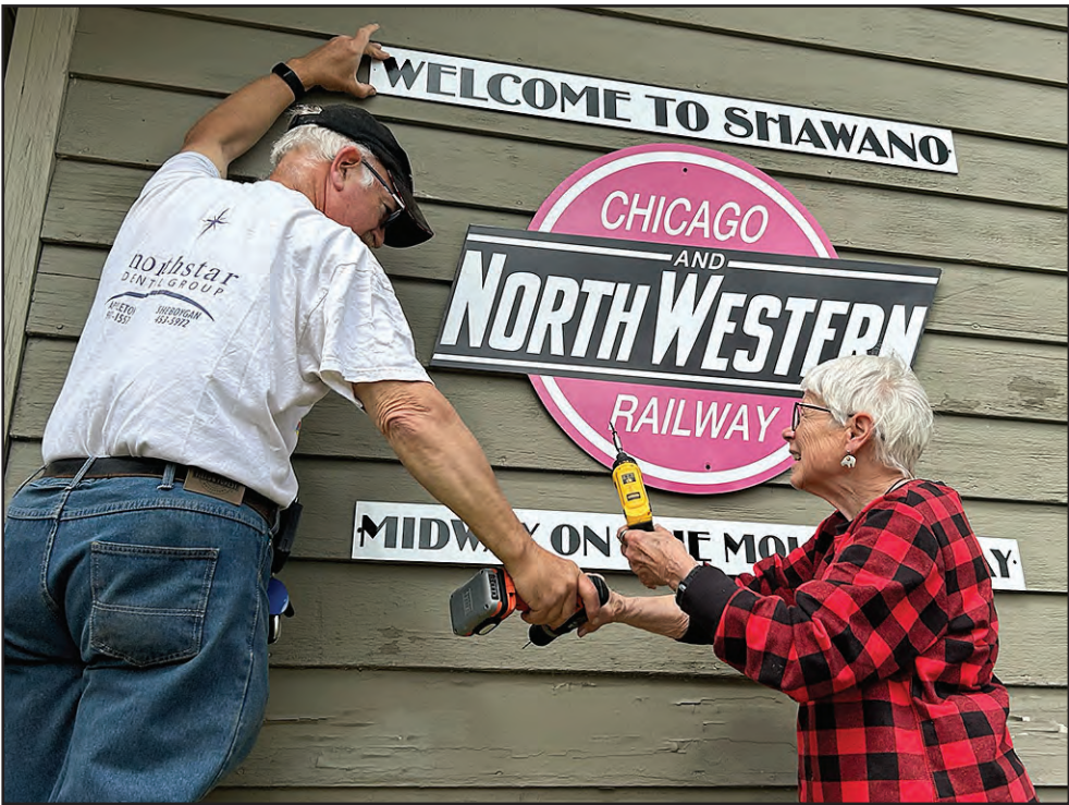
Kevin King and Matty Mathison install signs on the east side of the new Midway on the Mountain-Bay Trail Information Center, a former Chicago and Northwestern depot. The center has been a joint project of Friends of the Mountain-Bay Trail — Shawano County and Shawano Pathways.
