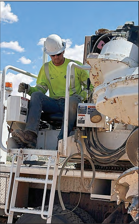
Central Wisconsin Electric Cooperative lineman Josh Wick operates a pressure digger. Most of the pole holes required a pressure digger because of rock in the area.
