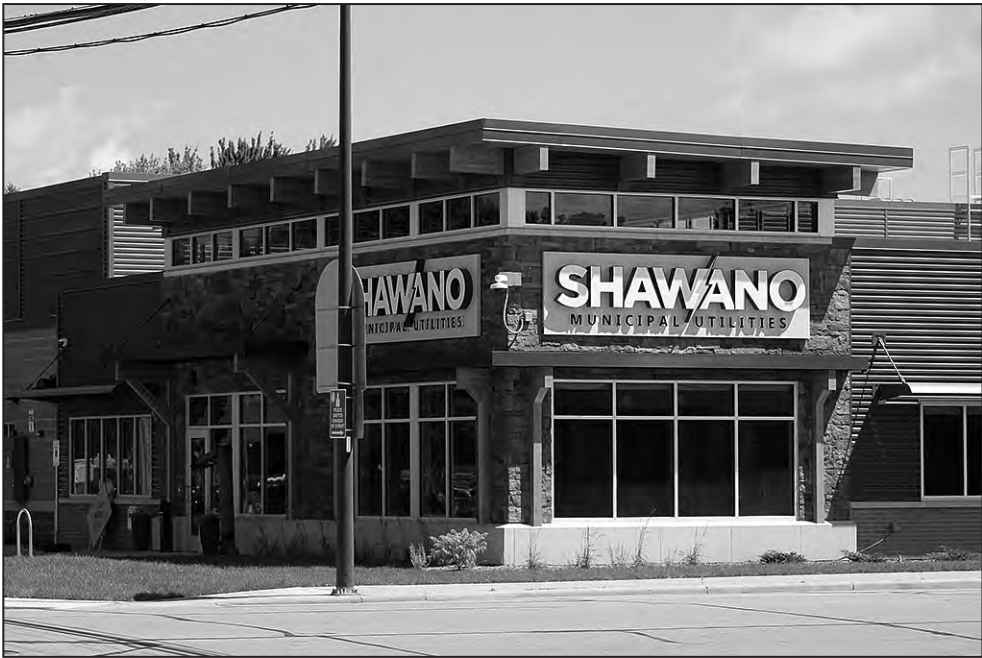
The new Shawano Municipal Utilities building at the corner of Green Bay and Sawyer streets opened almost two months ahead of schedule, modernizing how the utility does business.
