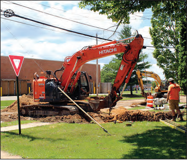
Crews work on Fifth Street between Hamlin and Union streets the afternoon of June 26. East Fifth Street from North Main Street to Hamlin Street is undergoing utility work and street reconstruction.
