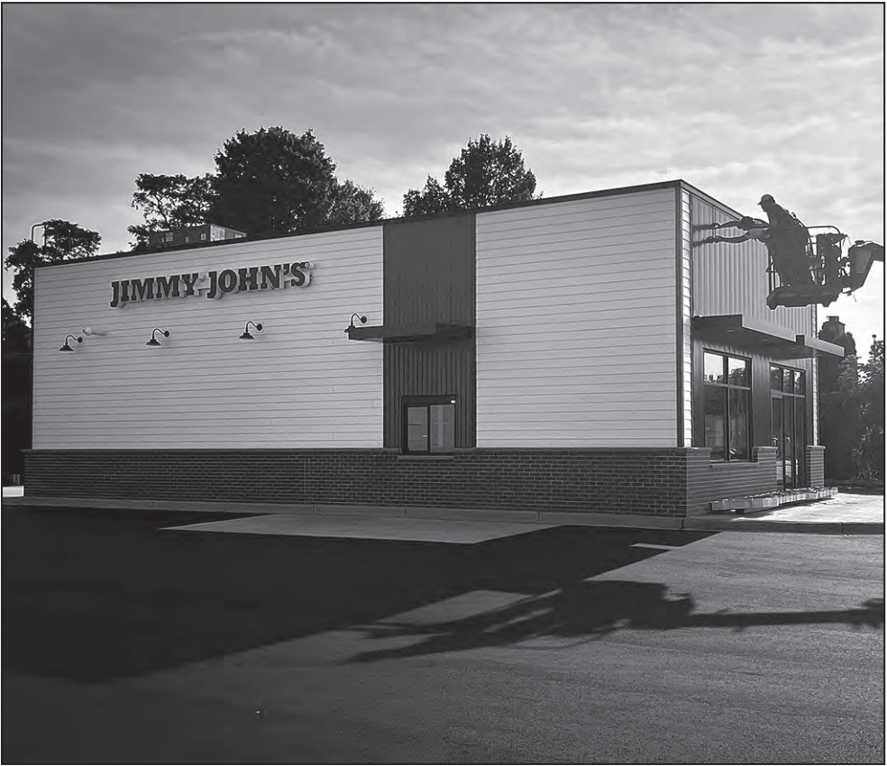
Workers at the new Jimmy John's, 811 E. Green Bay St., Shawano, continue their progress on the exterior of the restaurant. The new restaurant will include a drive-thru. Open job interviews were held July 29, while an official opening date has yet to be announced.
