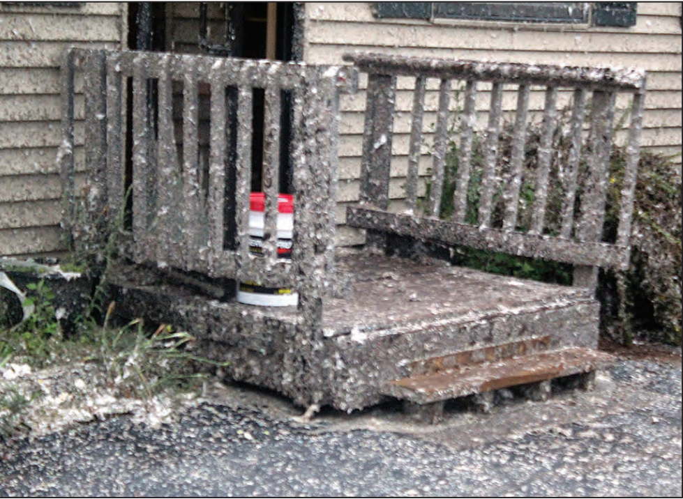
Debris still covers the entryway to Telford Equipment Consulting Co. in Gillett on July 24 following a storm that caused damage in Menominee and Oconto counties.
