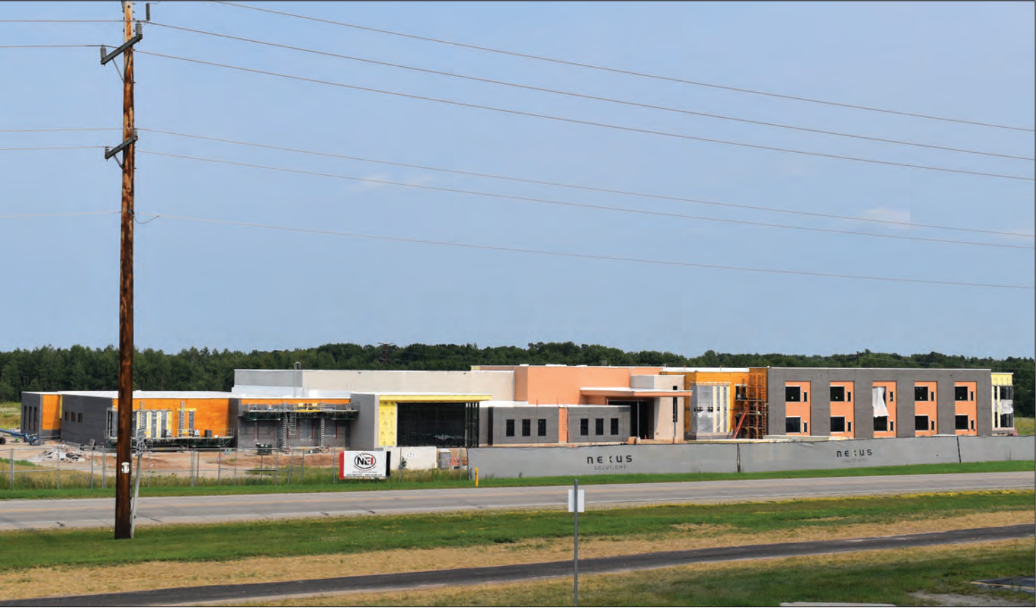
Work proceeds on schedule for the new Oconto Falls Middle School under construction along County Road I. WARREN BLUHM | NEW MEDIA
