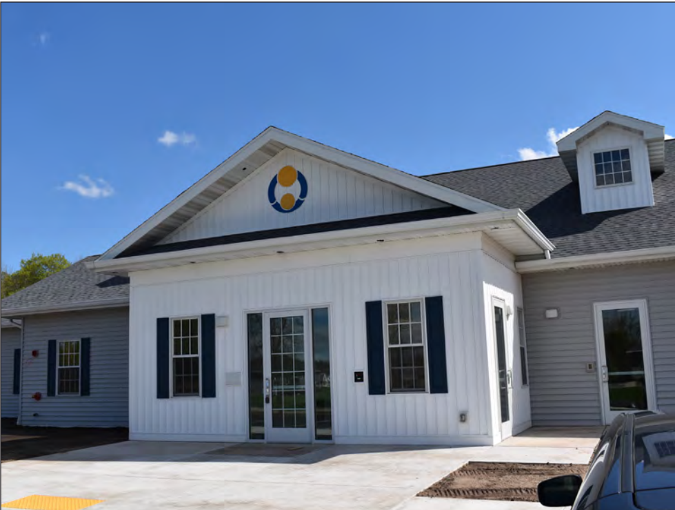
The new Encompass Early Education and Care Center in Oconto Falls was constructed on the bones of the former Kaempfer and Associates engineering office. The only addition to the building is the vestibule at the front. WARREN BLUHM | NEW MEDIA
