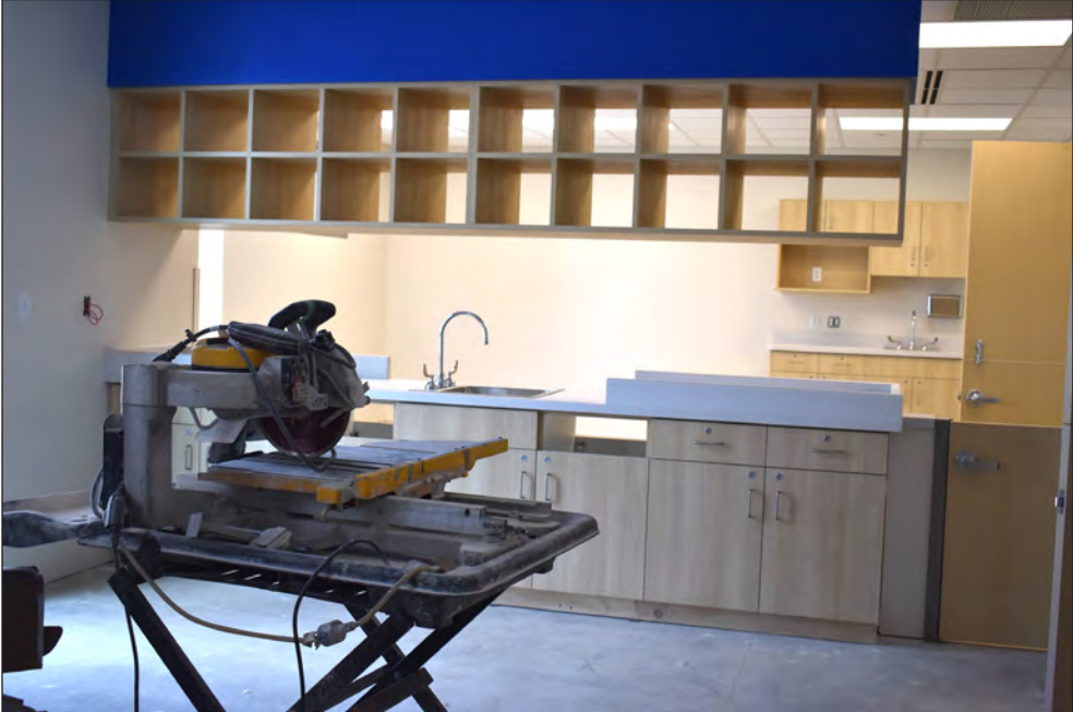
There’s still work to be done, but the infants rooms at the new Encompass Early Education and Care Center in Oconto Falls is taking shape May 8, a little more than a month before the facility at 650 Jackson St. is scheduled to open. WARREN BLUHM | NEW MEDIA
