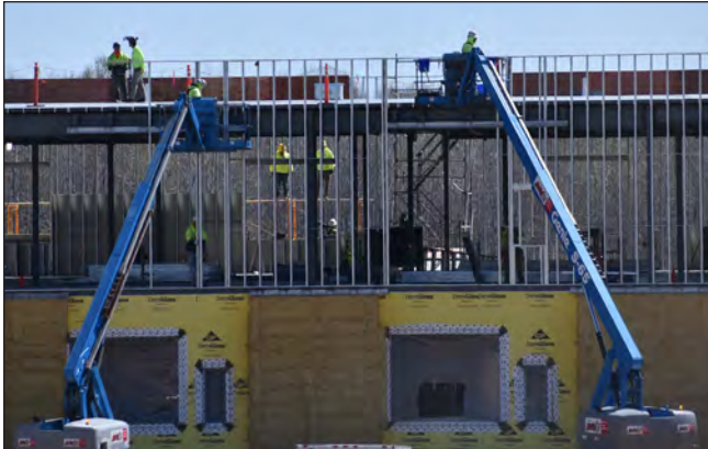
Steelwork is completed for the entire building, rubber roofing over the new gymnasium is installed, and exterior framing, underground plumbing, and electrical work continues.
