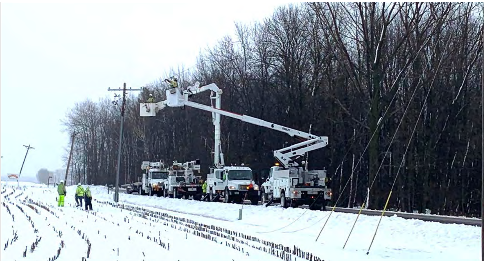
Oconto Electric Cooperative crews work to restore power to a large area of Oconto County on April 3.
