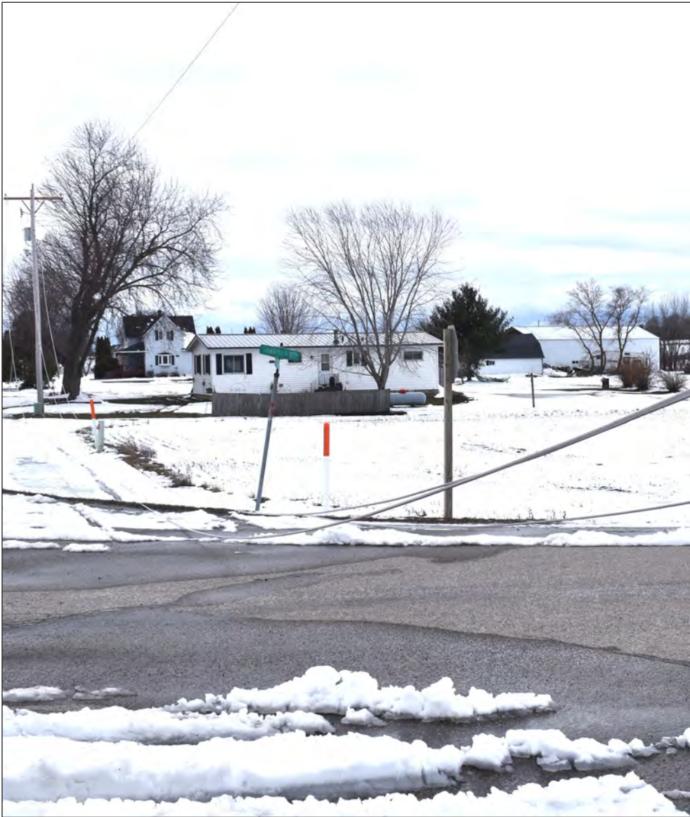
Newly strung electric cables droop across Belgian Road at the intersection with County Road A in the Town of Lena on April 4.
