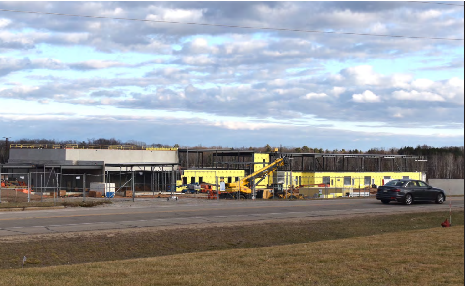
The frame of the new Oconto Falls Middle School can be seen March 19, and walls are being erected at the site along County Road I across from the high school. WARREN BLUHM | NEW MEDIA
