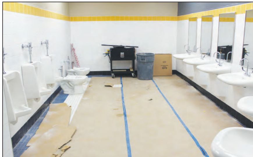
New bathroom facilities adjacent to the gymnasium are still being worked on, but Bonduel School District officials expect everything to be ready by the May 15 opening.
