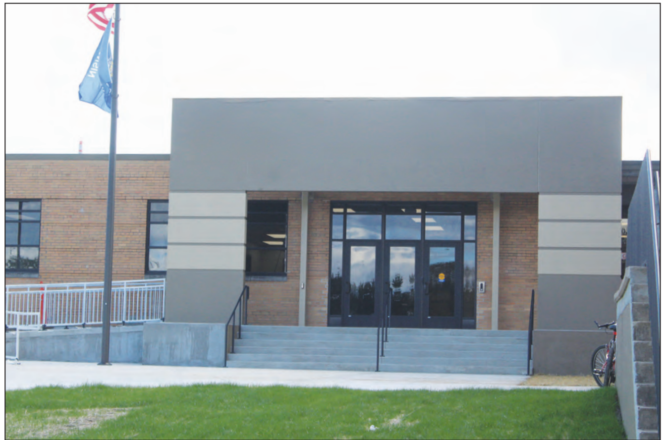
Bonduel Middle-High School has a new entrance that was completed over the summer, but signage still needs to be completed. LEE PULASKI | NEW MEDIA
