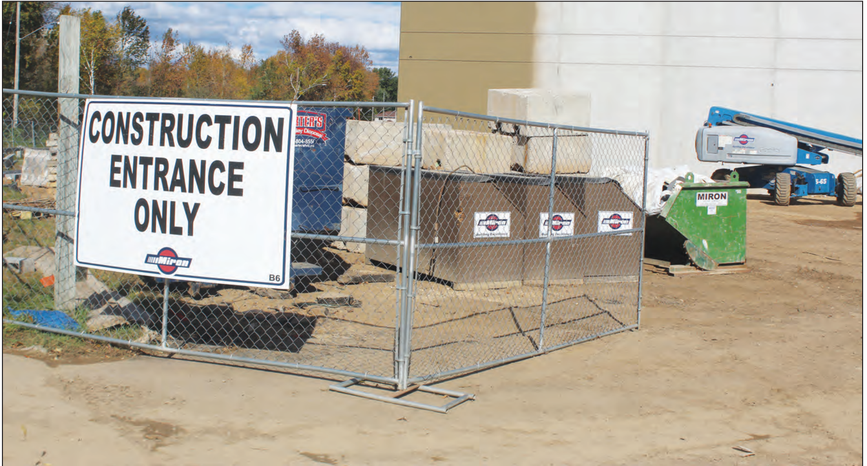
The walls are being put up on the new gymnasium for Bonduel Middle-High School, which is taking up the old parking lot area. Parking has been set up closer to Green Bay Street.
