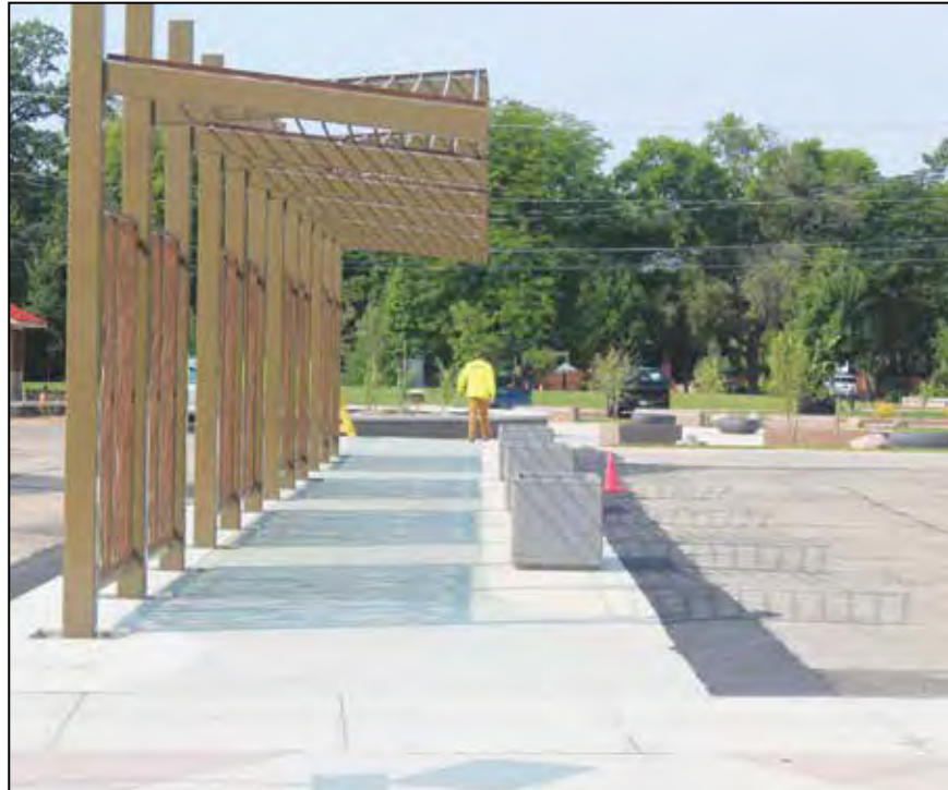
The plaza for downtown Shawano is complete except for lighting and installation of the fire feature, which are delayed by a few weeks. The plaza is open for public use and will be a part of the downtown Oktoberfest next week and the city's tree display with Franklin Park in November.
