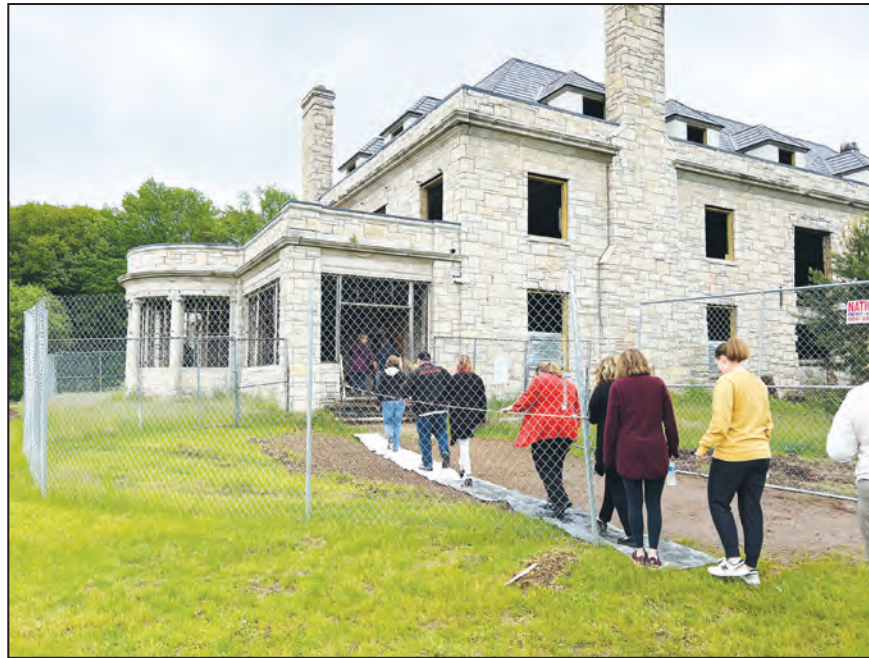
Shawano Rotary Club members walk the trail to enter the Alexian Brothers Novitiate on June 6. The Novitiate is currently undergoing roofing repairs, with other damage from a 1975 standoff looking to be renovated.
