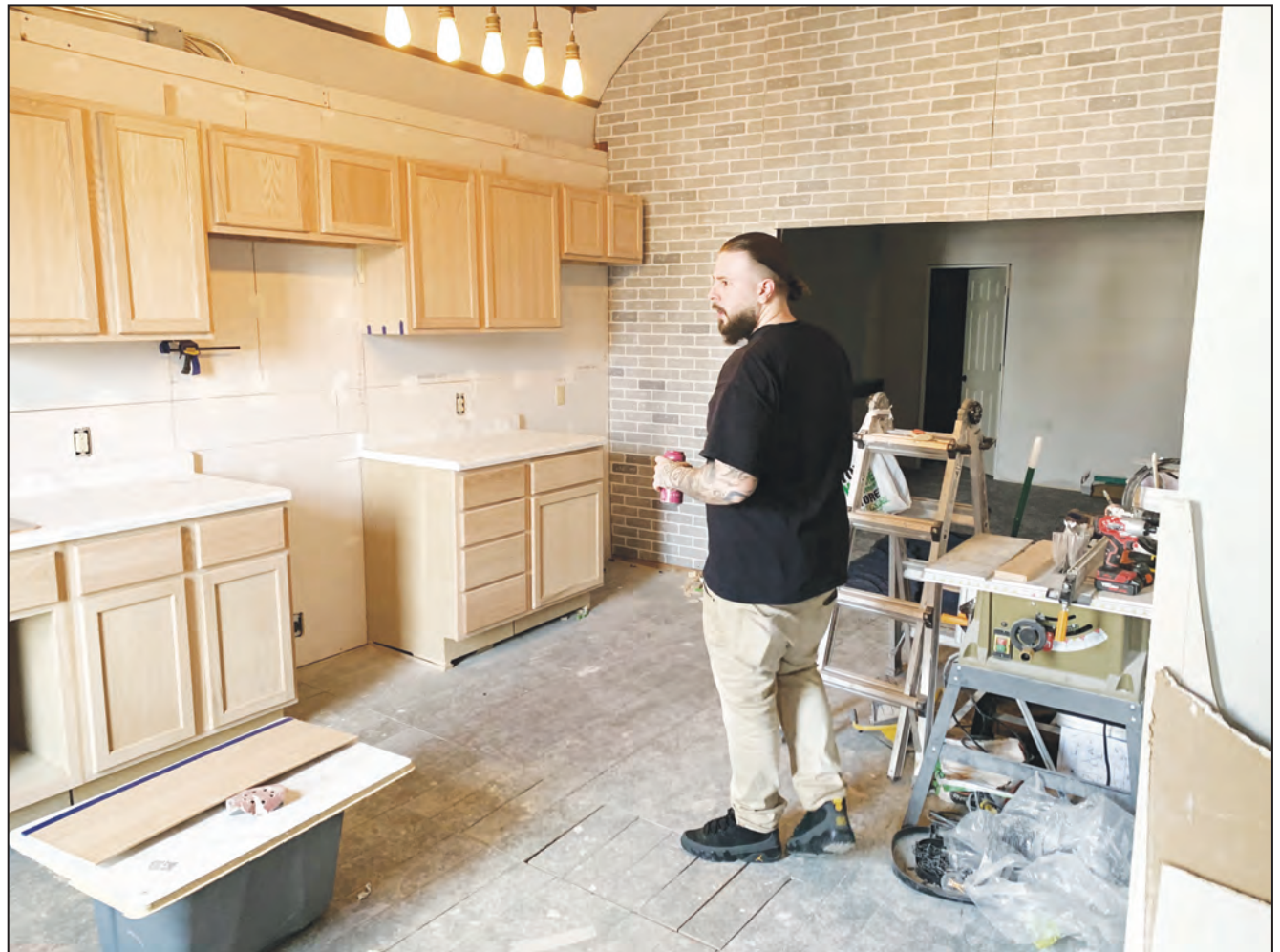
The Shawano Barbers owner Jesse Krajenka works through the renovations in the upstairs area of the barbershop. He is working on renovating the upstairs into a living quarters. LUKE REIMER | NEW MEDIA
