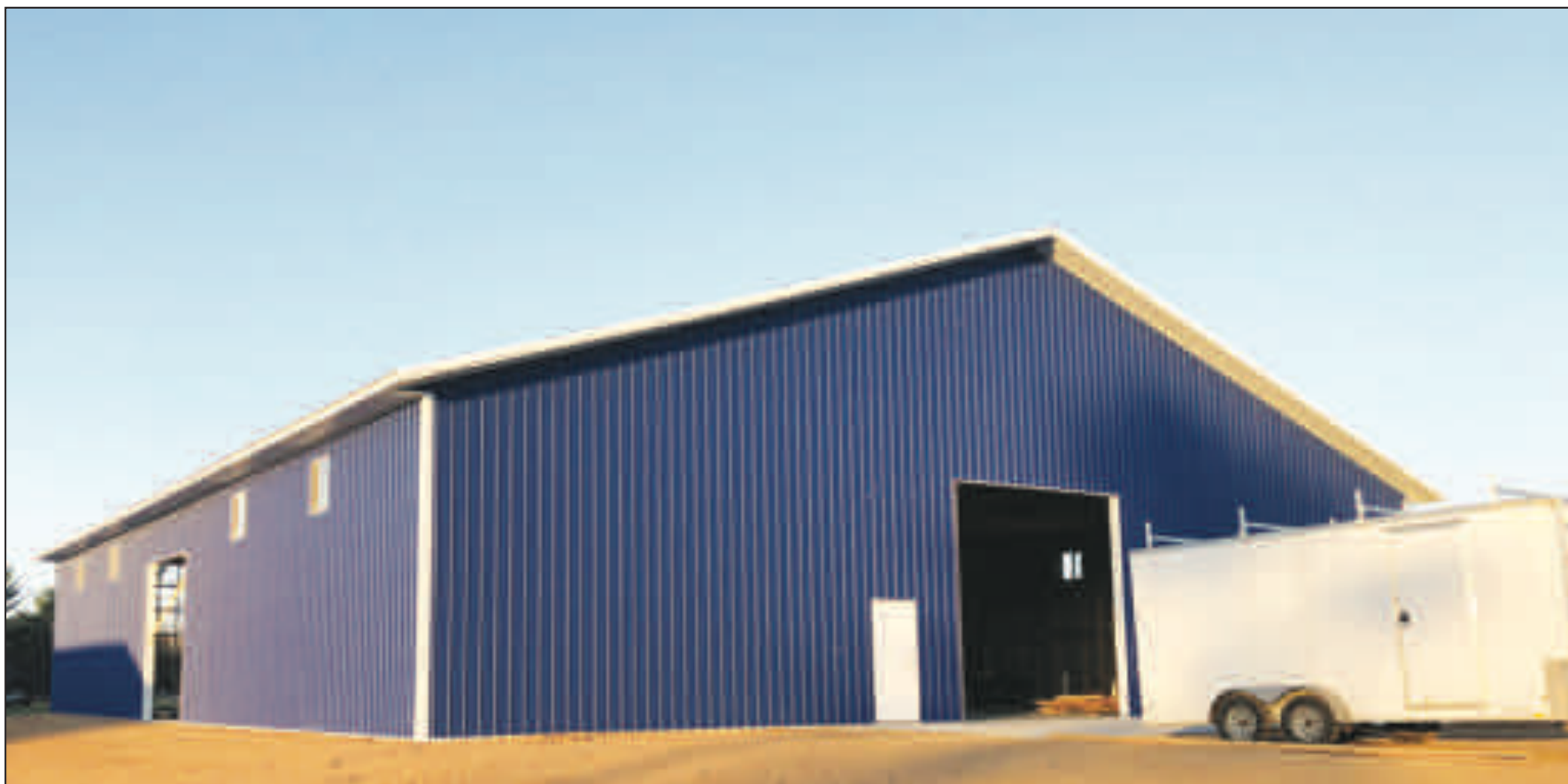
A red roof, blue siding and white trim of the new warehouse will echo the color scheme of the Fireworks Country retail space, west of Wittenberg. By the end of the week the exterior and interior of the warehouse should be finished.
