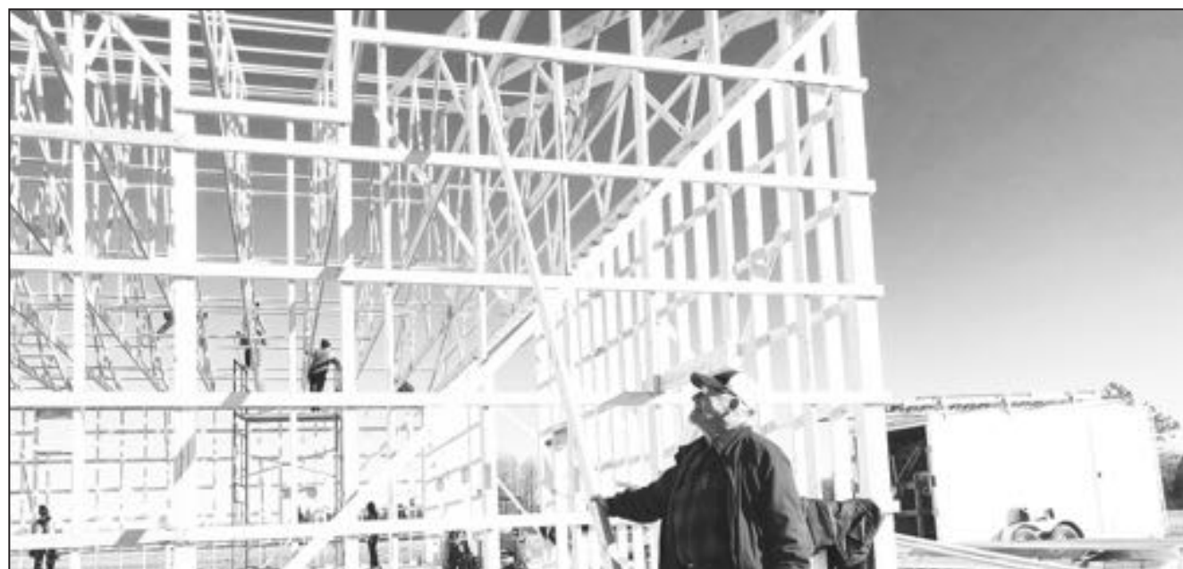
Paul Ostrowski Cement & Mason poured the six inches of concrete and Kauffman Carpentry did the framework of the new warehouse building at Fireworks Country, Wittenberg
