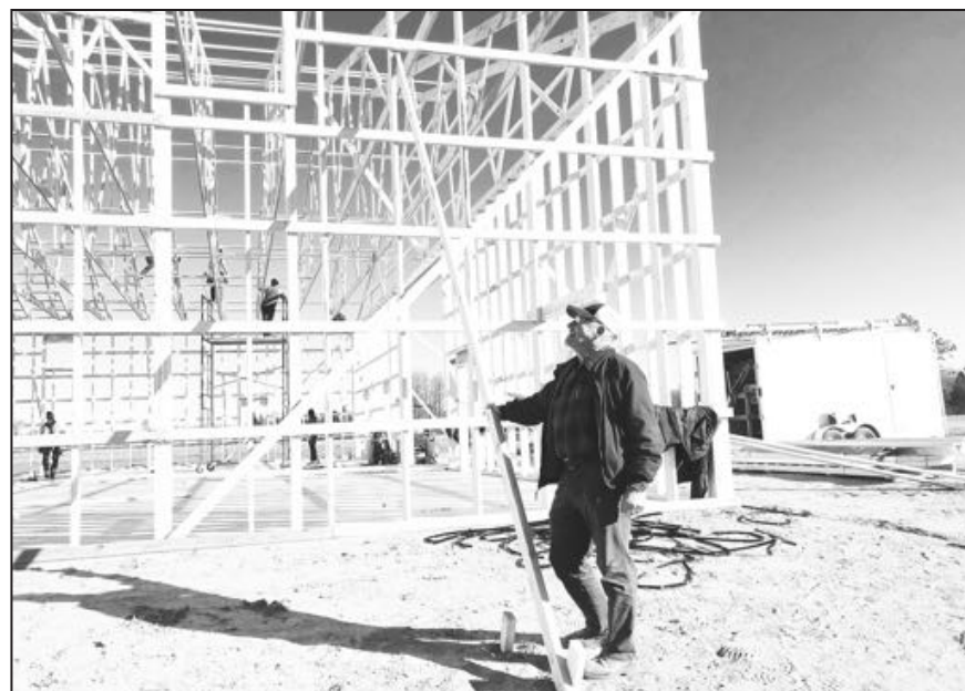
Jerry Bamke, owner of Fireworks Country, Wittenberg, inspects the framing being done by Kauffman Carpentry, Marion, for his new 8,000 square foot warehouse.
