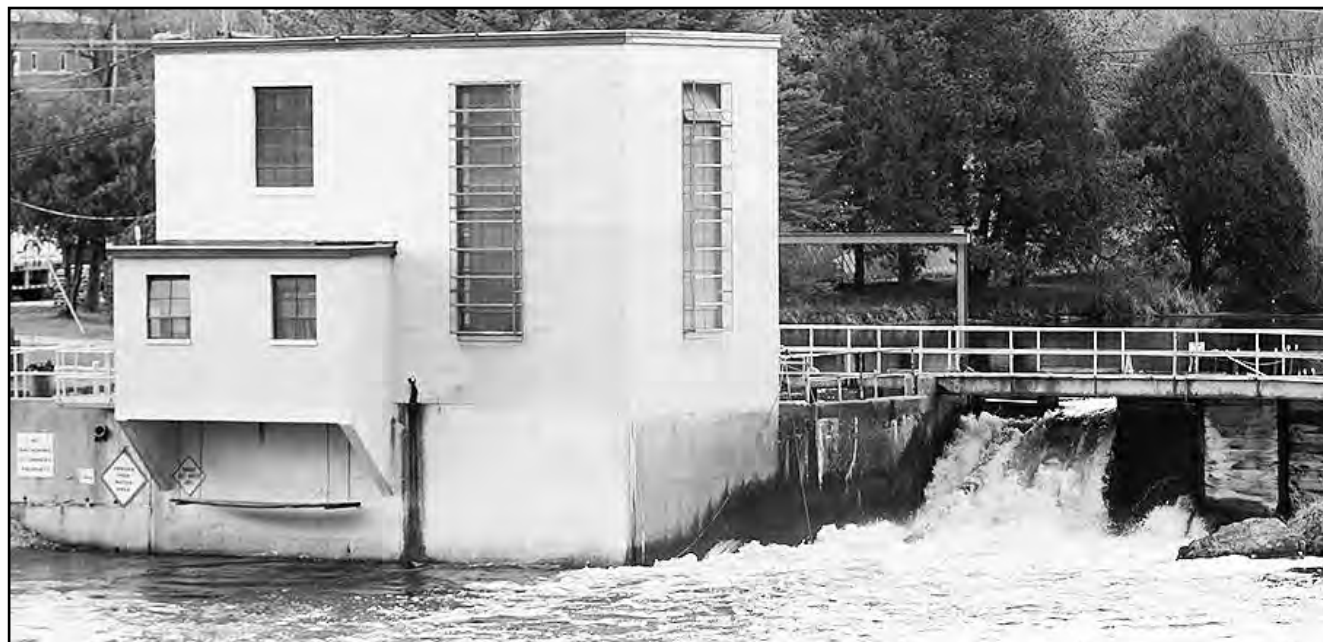
The spillways at the Shawano Paper Mill dam allows operators to control the water flow and the level of water upstream. An effort is underway by the Shawano Area Waterways Management (SAWM) to maintain water levels at 802.9 feet above sea level all year-round.
