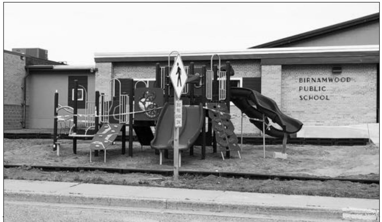
The new handicapped accessible entrance and classroom additions are nearing completion at the Birnamwood Elementary-Middle School, located at 337 Main St., Birnamwood.
