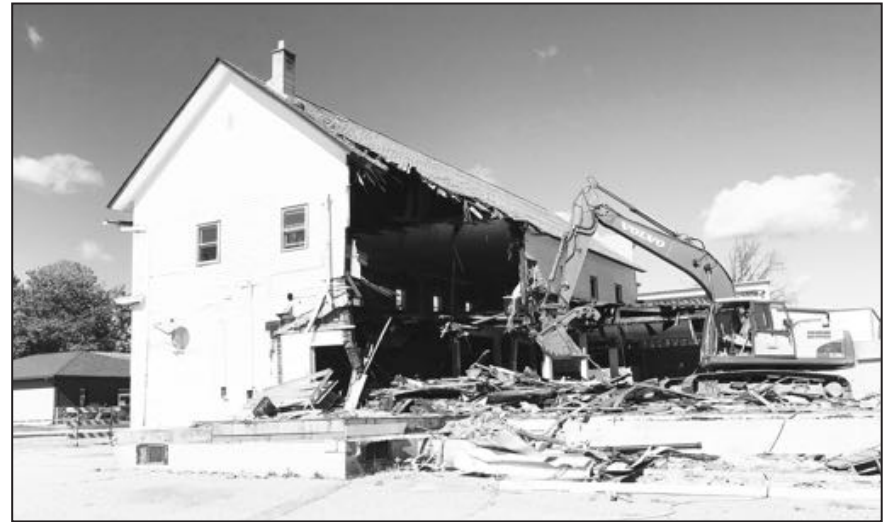
Jack Kautza has been demolishing buildings for 50 years. His company, Kautza Excavating LLC, tore down the former Backes Food Mart building in downtown Birnamwood in 8-10 hours.
