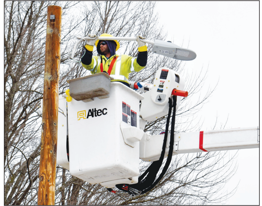
John Bestul, service foreman for Central Wisconsin Electric Cooperative, installs a new LED light fixture to a light pole in the village of Tigerton.
