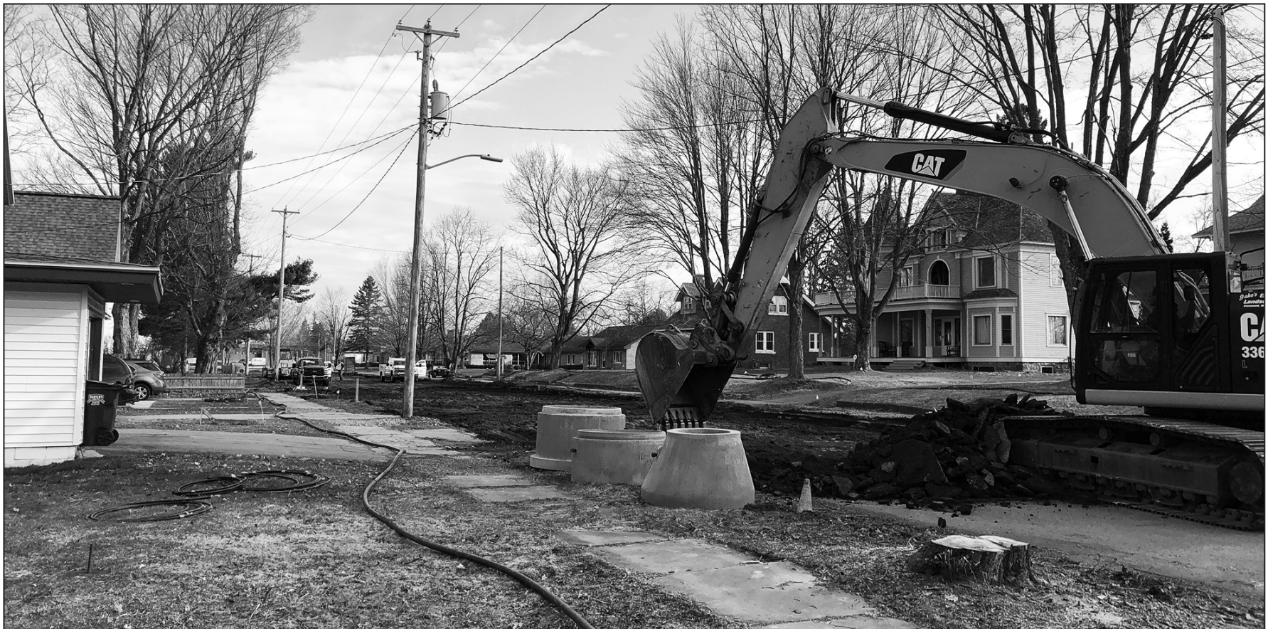
The trees are down, the asphalt being removed and life on Webb Street will be interesting for those who live there. The project is expected to be finished before the end of May. MIRIAM NELSON | NEW MEDIA
