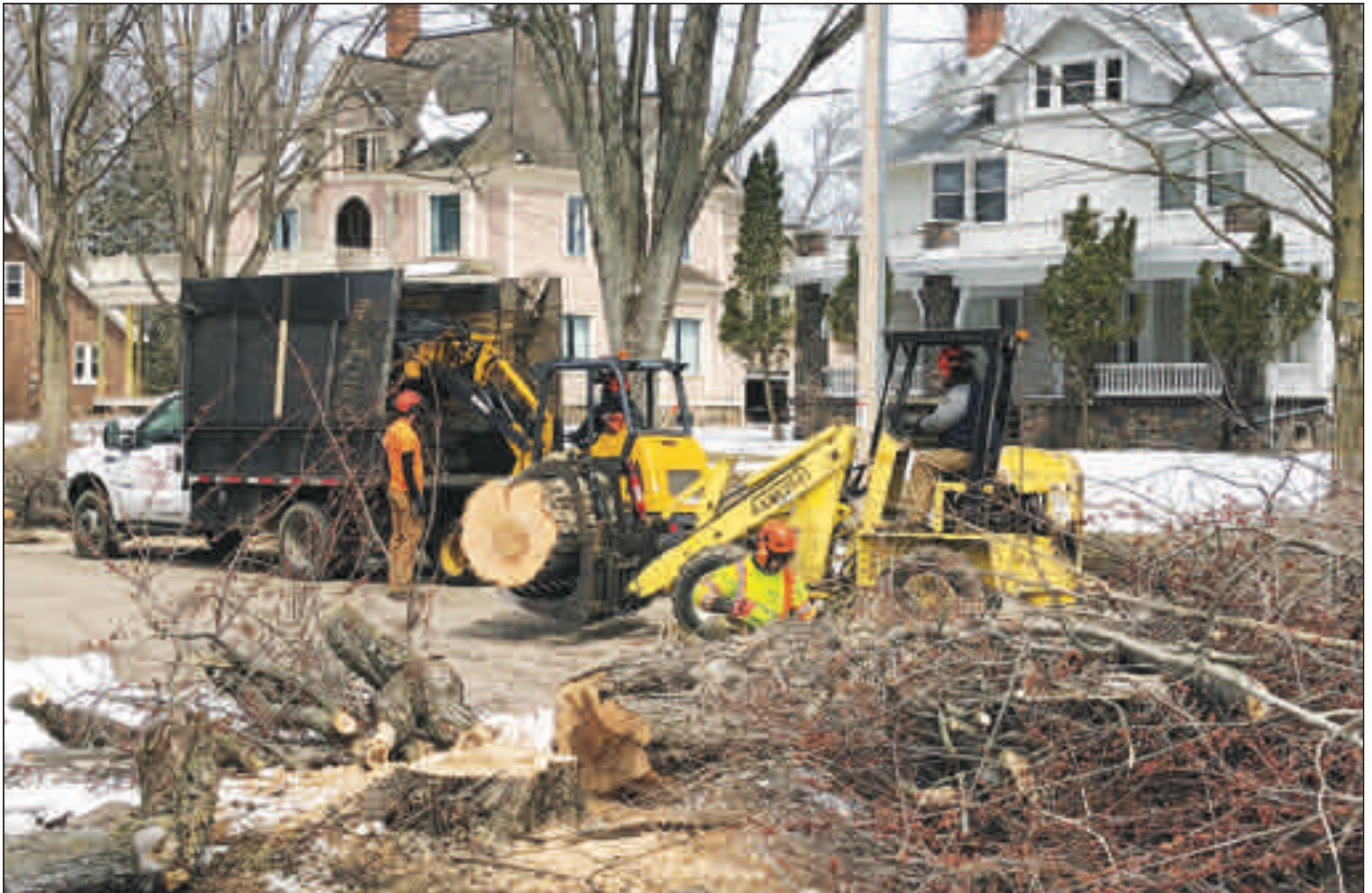
Tree Fella, of Wausau, cuts down 25 trees April 15 in preparation for the Webb Street reconstruction project. The road work on the street, curbs and gutters is scheduled to begin in May.
