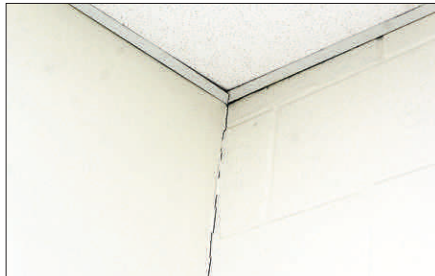
Cracks and decay are appearing at various spots at Bonduel High School. The Bonduel School District is hoping to modernize the school, if voters approve a $12.5 million referendum in April.
