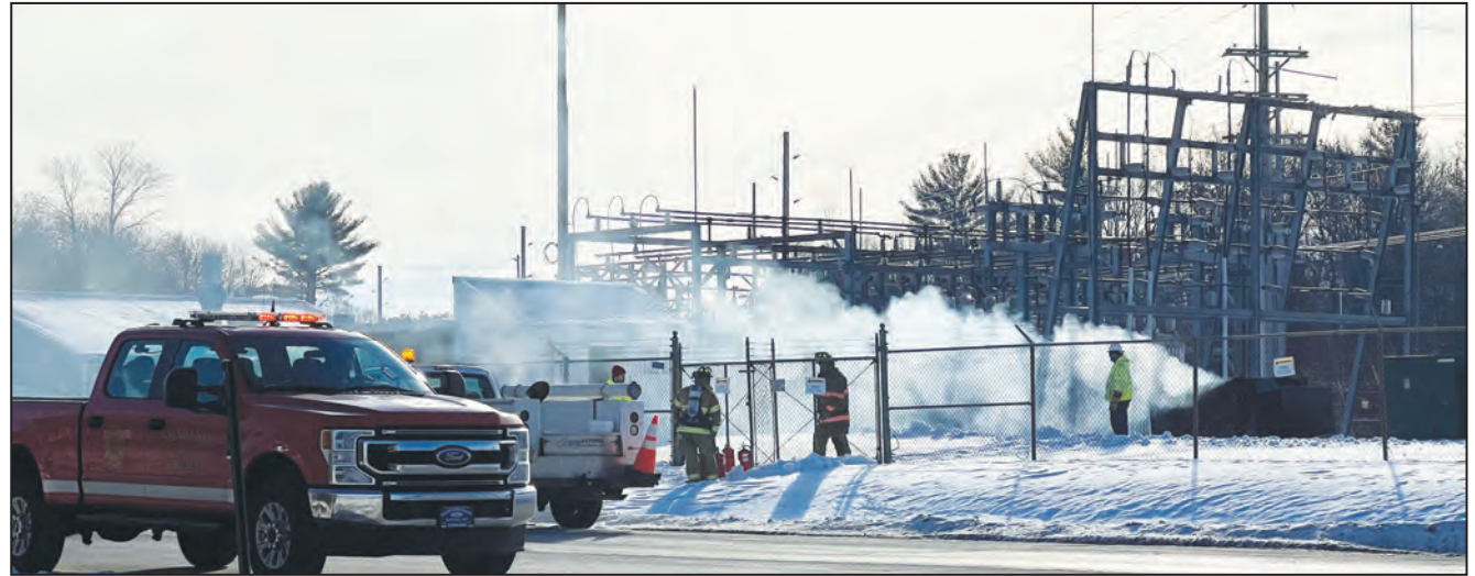
Crews with Shawano Area Fire Department work to put a fire at one of the city’s industrial substations on Feb. 1. The fire occurred after an equipment failure, said Shawano Municipal Utilities General Manager Bruce Gomm. He added that when SMU switched directions of power, a fault was fed and the back feed from the fault caused the fire.
