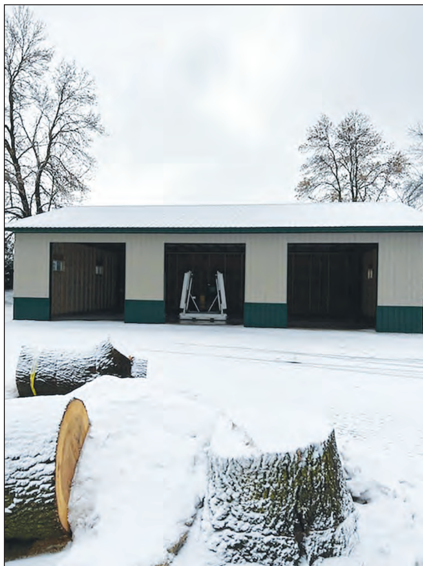
A new building is waiting for garage doors to be placed on it at the Shawano County Fairgrounds. The new building was constructed to house bingo during the Shawano County Fair, something that Shawano Speedway and Fairgrounds Marketing and Promotions Manager Brad Luepke said would be an improvement over holding it under a tent.
