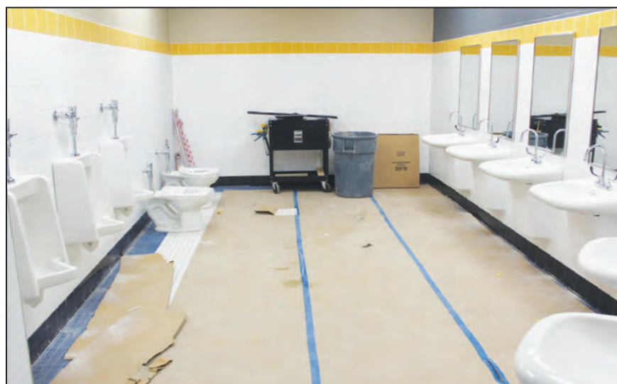
New bathroom facilities adjacent to the gymnasium are still being worked on, but Bonduel School District officials expect everything to be ready by the May 15 opening.
