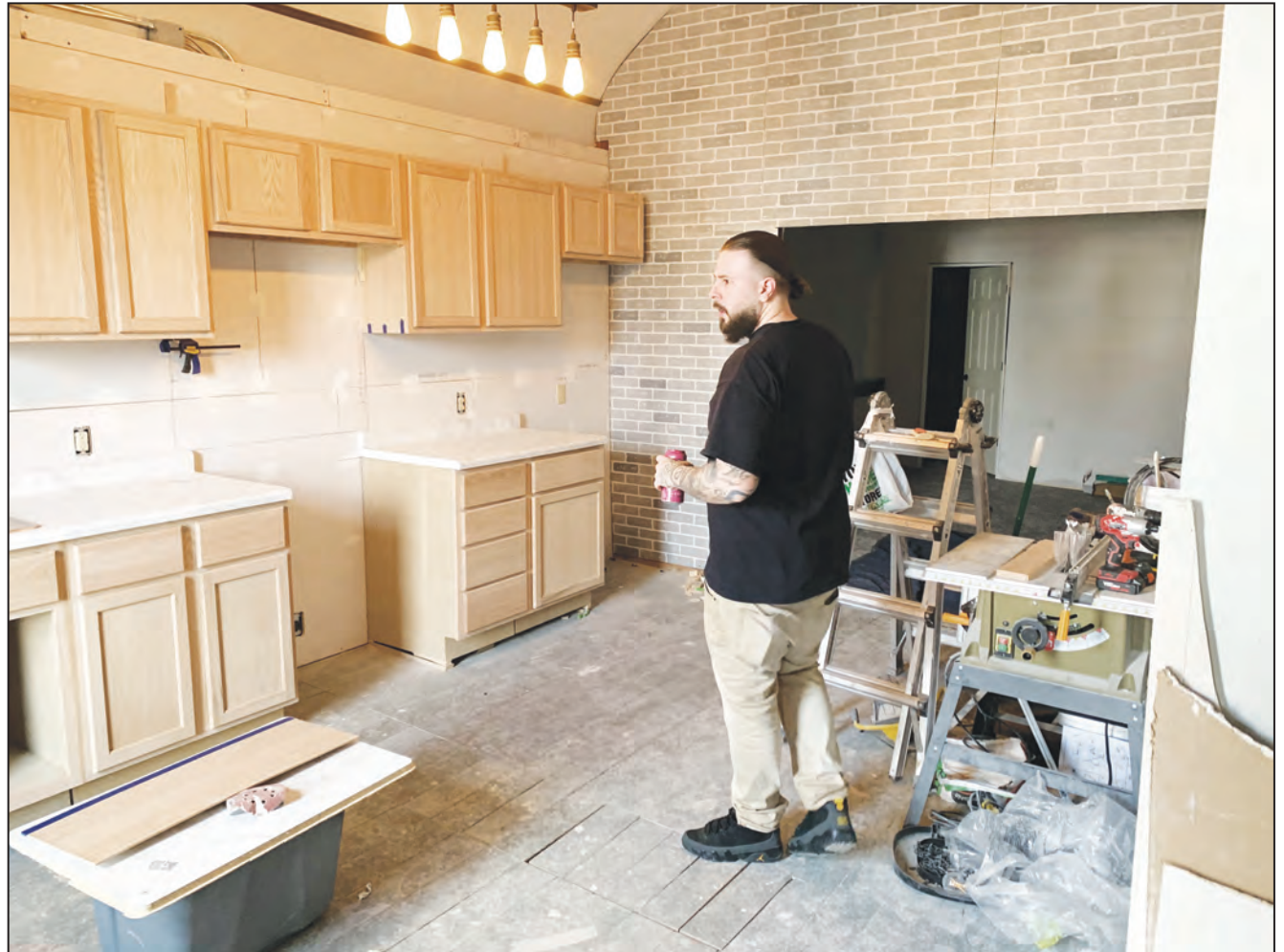
The Shawano Barbers owner Jesse Krajenka works through the renovations in the upstairs area of the barbershop. He is working on renovating the upstairs into a living quarters.
