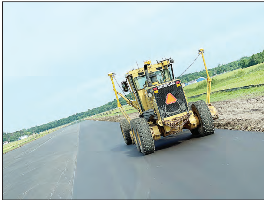
Shawano Airport runway 1230 continues to be repaved in order to fill cracks and keep up with asphalt life. The project is expected to finish on the weekend of July 4.
