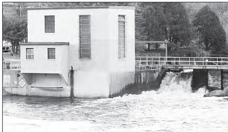
The spillways at the Shawano Paper Mill dam allows operators to control the water flow and the level of water upstream. An effort is underway by the Shawano Area Waterways Management (SAWM) to maintain water levels at 802.9 feet above sea level all year-round.
