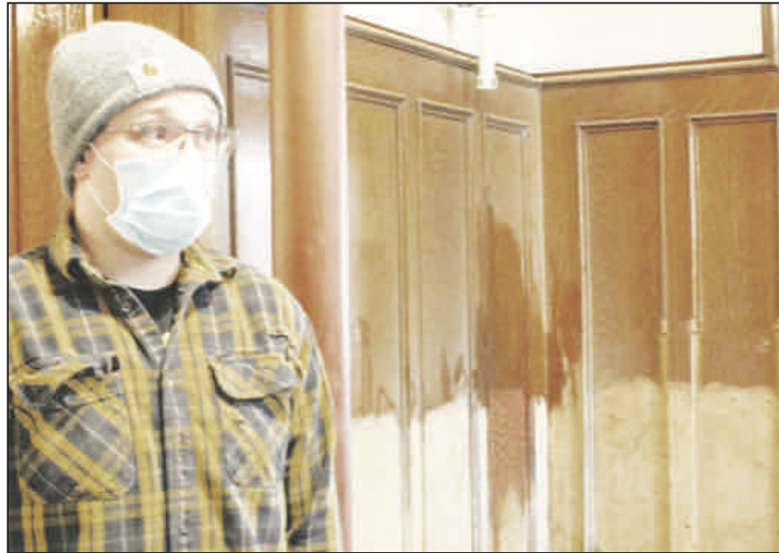
Aaron Damrau pauses in his restoration work at the Swanke mansion in Tigerton. He's standing near some of the oak woodwork in the entryway that's being refinished. Herman Swanke used generously the wood and millwork produced in his Tigerton Lumber Company in building the home in 1920.
