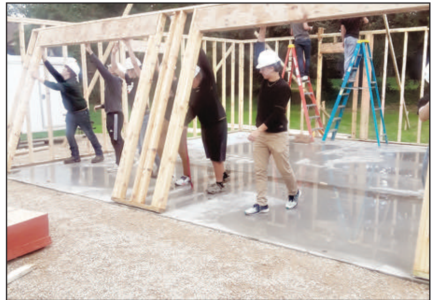
Clintonville High School students are constructing a 24-by-24-foot two-car garage for the rental property owned by Dan Gehrke in Clintonville. The junior and senior students participating in construction classes at the school are learning all the carpentry skills necessary to work in the construction industry, including framing, siding, roofing and design.
