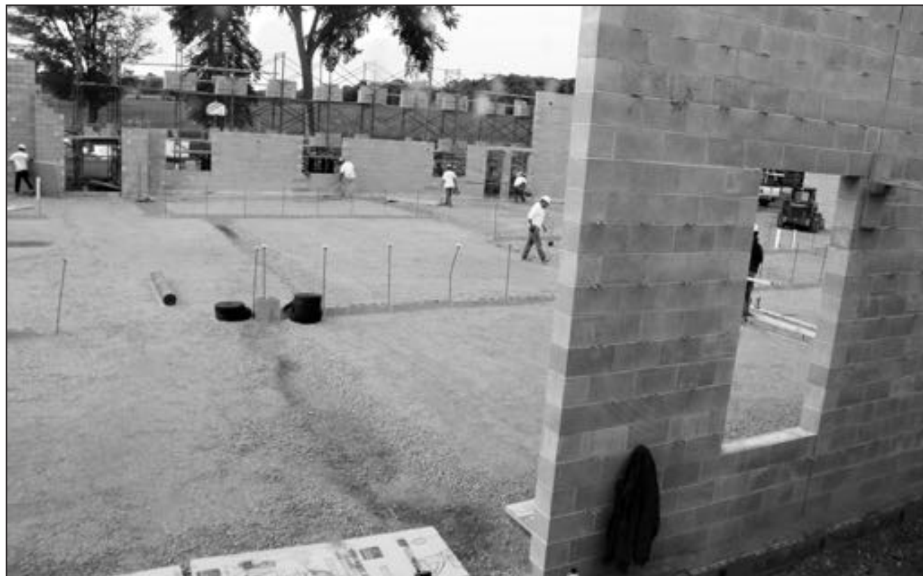
A view from the second floor of the current Gresham Community School shows employees from Kraus Anderson building the perimeter of the new middle school and high school sections Friday. Gresham school staff said that Kraus Anderson has brought in additional help when other projects were canceled to move construction a little ahead of schedule.
