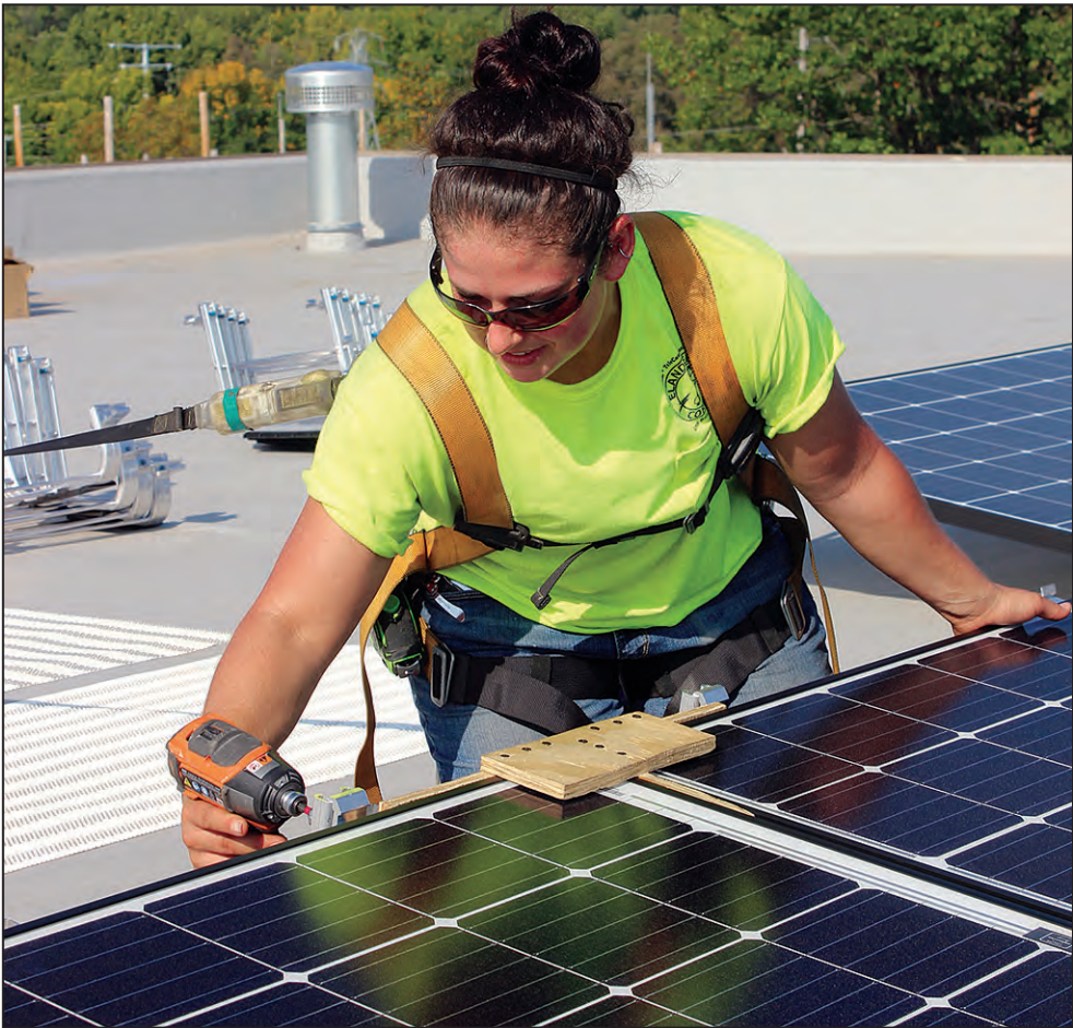
A Northeast Wisconsin Technical College student works on a solar panel.
