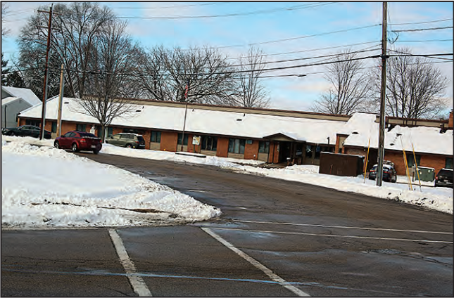
Fifth Street from Main to Hamlin will be one of the roads in Shawano undergoing reconstruction in 2024. Six segments of road will be replacing asphalt and adding sewer and water infrastructure, but Fifth Street will also be getting infrastructure for the city's storm sewer system.
