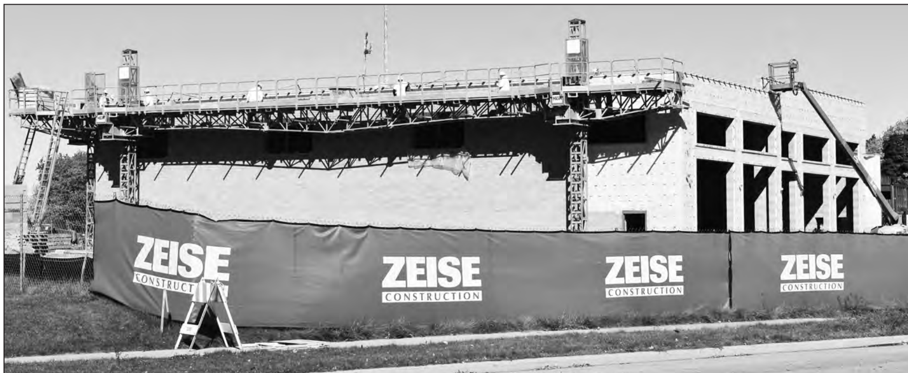
The new Oconto Falls Fire Department headquarters is beginning to take shape at the intersection where Columbia Street meets Union and South Chestnut avenues. The $7.5 million fire station, mostly funded by a federal grant, is scheduled for completion next summer.
