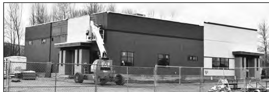
A work crew makes some finishing touches April 21 to the exterior of the New Beginnings retail store and training center on West Park Street in Gillett, which is expected to open later this spring.
