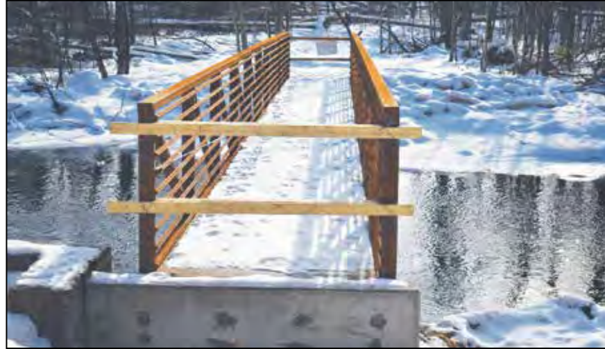
Approaches to the new Chute Pond Campground bridge will be built once the weather allows. A bathroom and new well at the Riverside campsites are on the 2022 work plan as part of the five-year Oconto County Parks and Recreation Plan.
