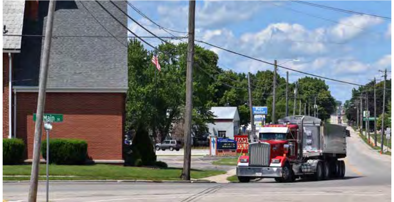
A 2026 reconstruction project is expected to bring state Highway 22 even closer to the "Clock Church," which brought some comment at a June 30 virtual meeting about the plan.
