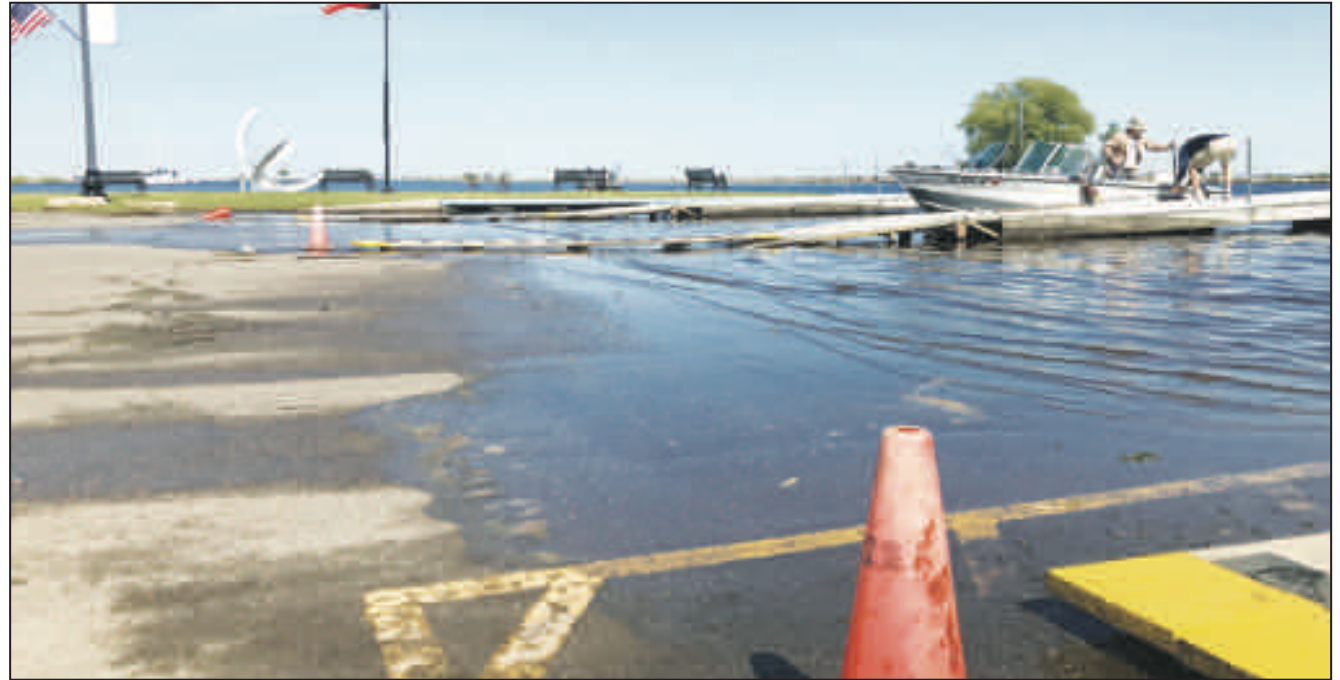
Boaters at the launch at Breakwater Park in Oconto have plenty of water to contend with. The U.S. Army Corps of Engineers expects levels to set another monthly record in August before starting to decline this fall.
